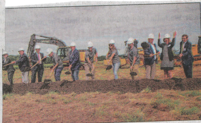
Oconee County and Impact Housing Group officials participated in a groundbreaking for the company’s planned complex at the Oconee Industry and Technology Park in Westminster on Tuesday.
