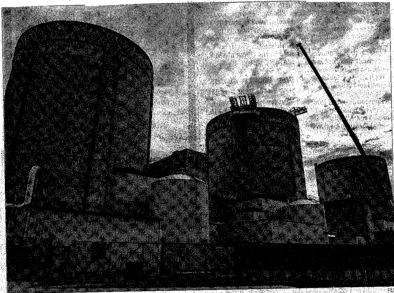
An Oconee Nuclear Station reactor was shut down after "an unusual event" early Saturday morning, according to a Duke Energy official. No one was injured. FILE
