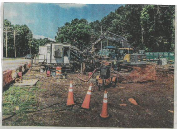
Construction equipment sits along Keowee School Road in Seneca. Existing electrical conduit along McMahon Bridge will be replaced with new runs, buried 15 feet under Lake Keowee.
