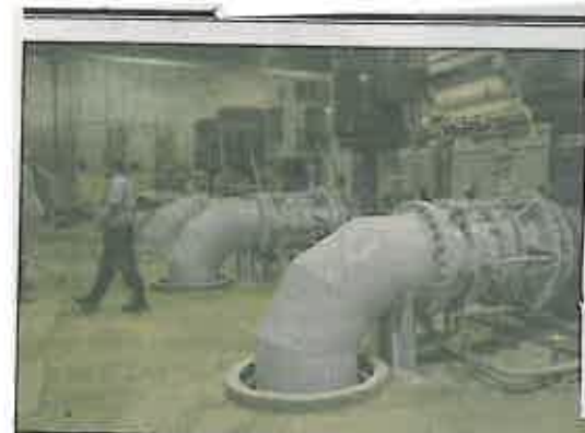
Water intakes on Lake Keowee draw 30 million gallons on an average day for the Greenville Water System. KEN OSBURN/STAFF
